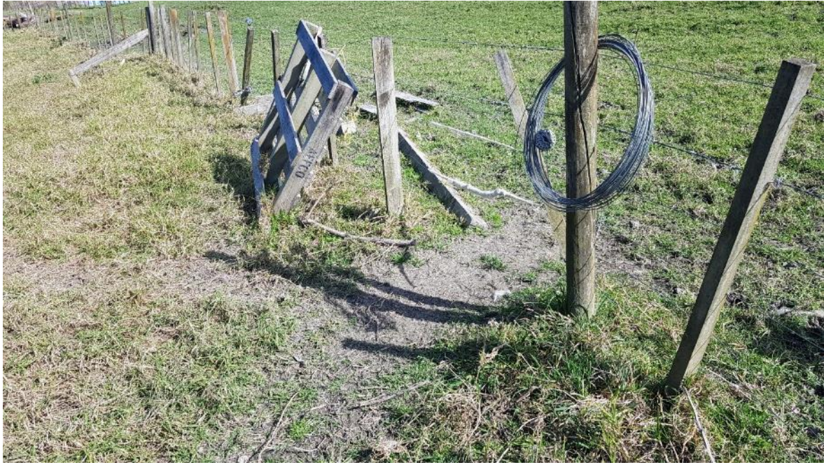
Figure 87. Inadequate fencing of the Awatere Stream inanga spawning site in Hawke’s Bay, September 2023. The fence had not been repaired by May 2024. (Photo: Mike Hickford)
