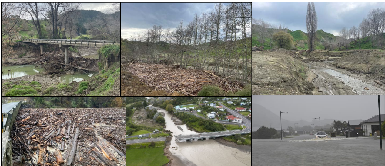
Figure 2 Photo mosaic of flood damage in Tairāwhiti (source: Thomas, 2024; NZ Herald, 2020)
